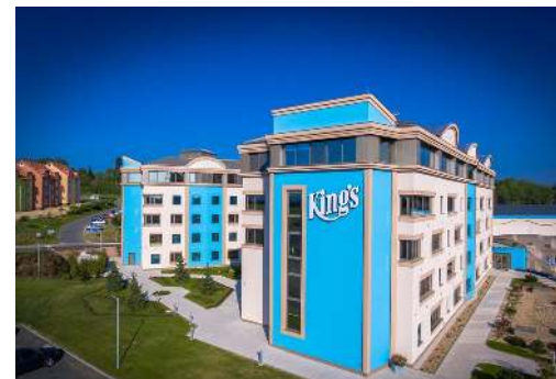
△ Hotel, Casino a Wellness King's, Rozvadov
