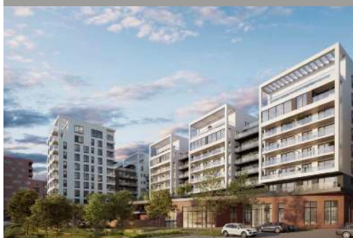
△ Daramis, Marina Island, Praha
